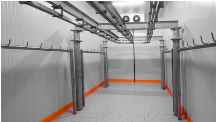
Cold Room and Storage
